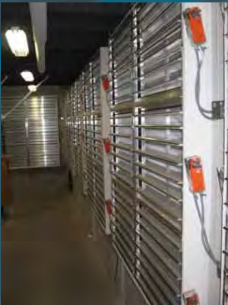
University of Sherbrooke Hospital Center Emergency Standby Generator Sherbrooke, Quebec.
